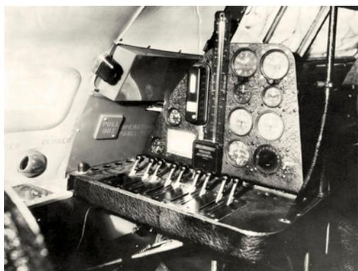
In June 1936, the War Department contracted with Lockheed to create a fast, high-altitude flier, the XC-35. During test flights, the plane reached a top speed of 350 mph, and the pressurized cabin made flight possible above 30,000 feet without the use of oxygen. The XC-35 earned the Collier Trophy for the most significant aircraft development of 1937.
