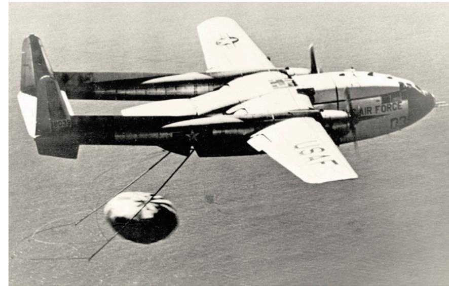
On August 19, 1960, the Discoverer/Corona 14 dropped its film from space. Once it entered the Earth’s atmosphere, a parachute deployed and the recovery capsule was caught midair at an altitude of 8,000 feet.
