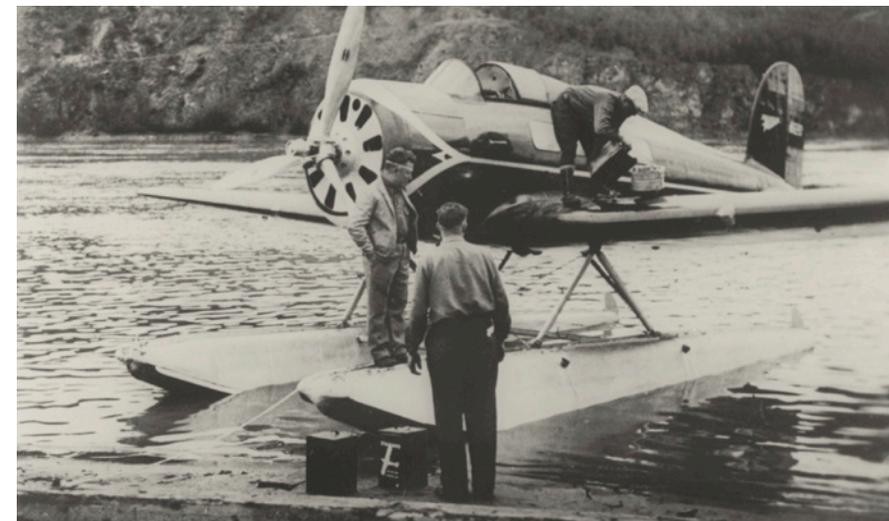
Wiley Post with his Orion-Explorer hybrid sea plane, which was built by mating the wing of Explorer 4 with an Orion 9E, 1935.
