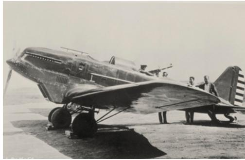
The XP-900/YP-24 was the first Lockheed fighter, first U.S. military monoplane fighter and first U.S. military aircraft with fully retractable landing gear, 1931.
