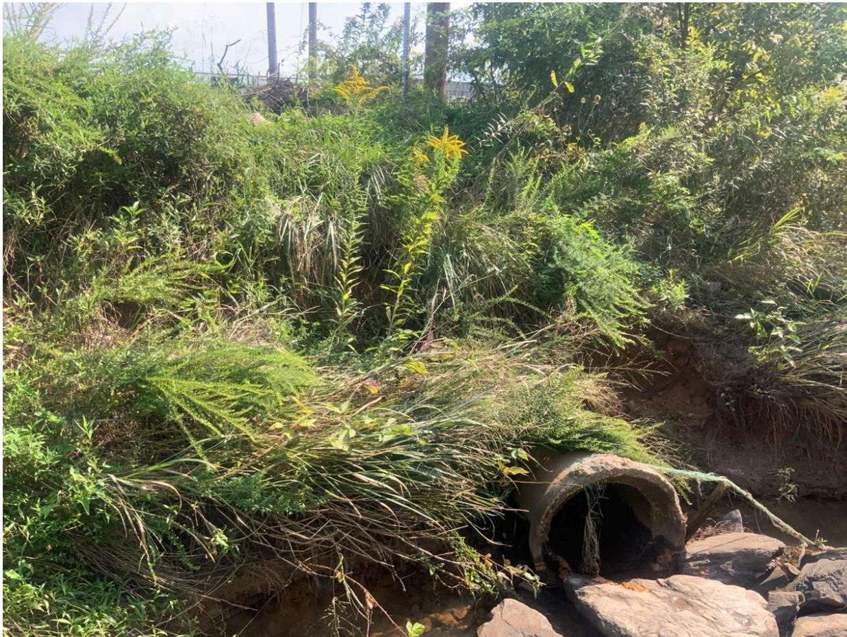
**Photo A-118.** Outfall pipe with erosion, left streambank at station 01+64, September 2021.
