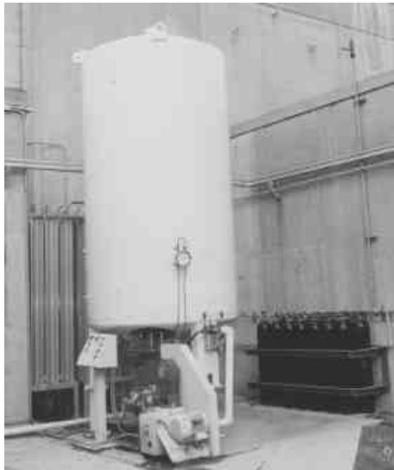
Figure 6-10 High Pressure Nitrogen Gas Facility
